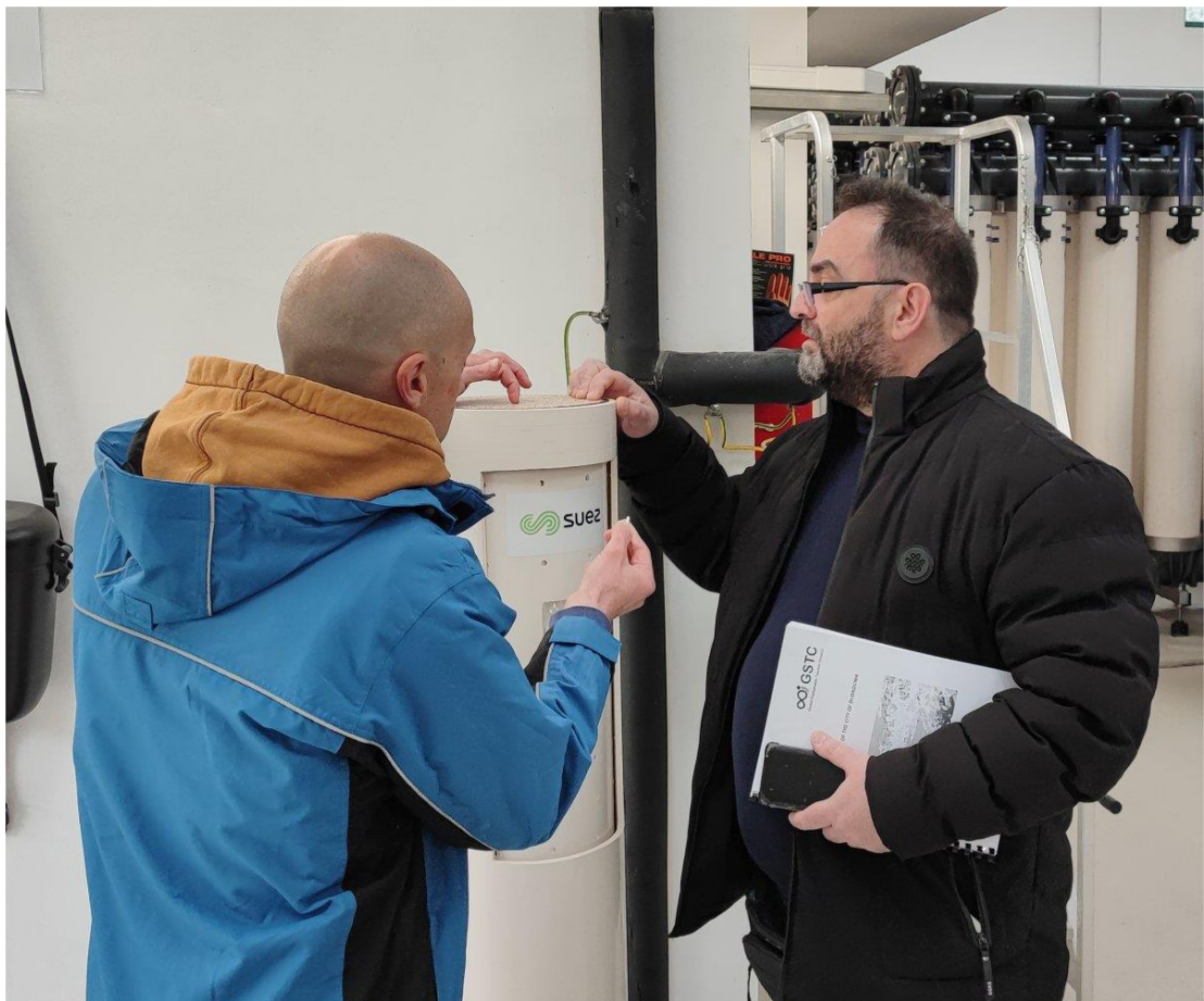
Figure 10: Field visit to Dubrovnik Water Facilities (Vodavod) in 2023
